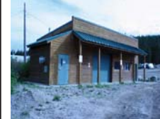
Main Water Plant
