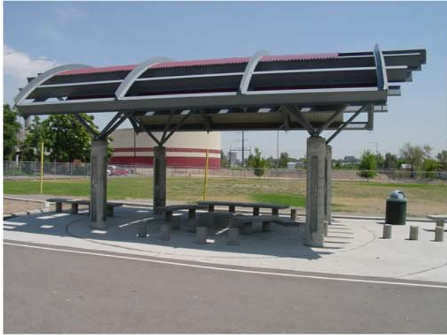
2001-10-09 VIEW shade structure.JPG
